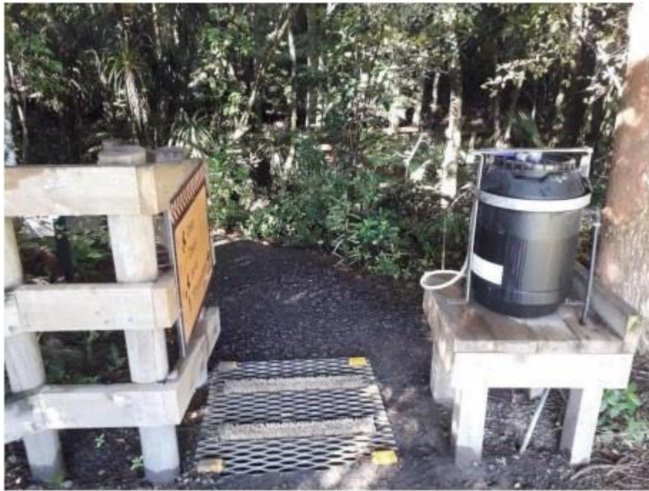
Figure 1.6 Barrel and grate wash station at Trounson park (Aley and MacDonald, 2018).
