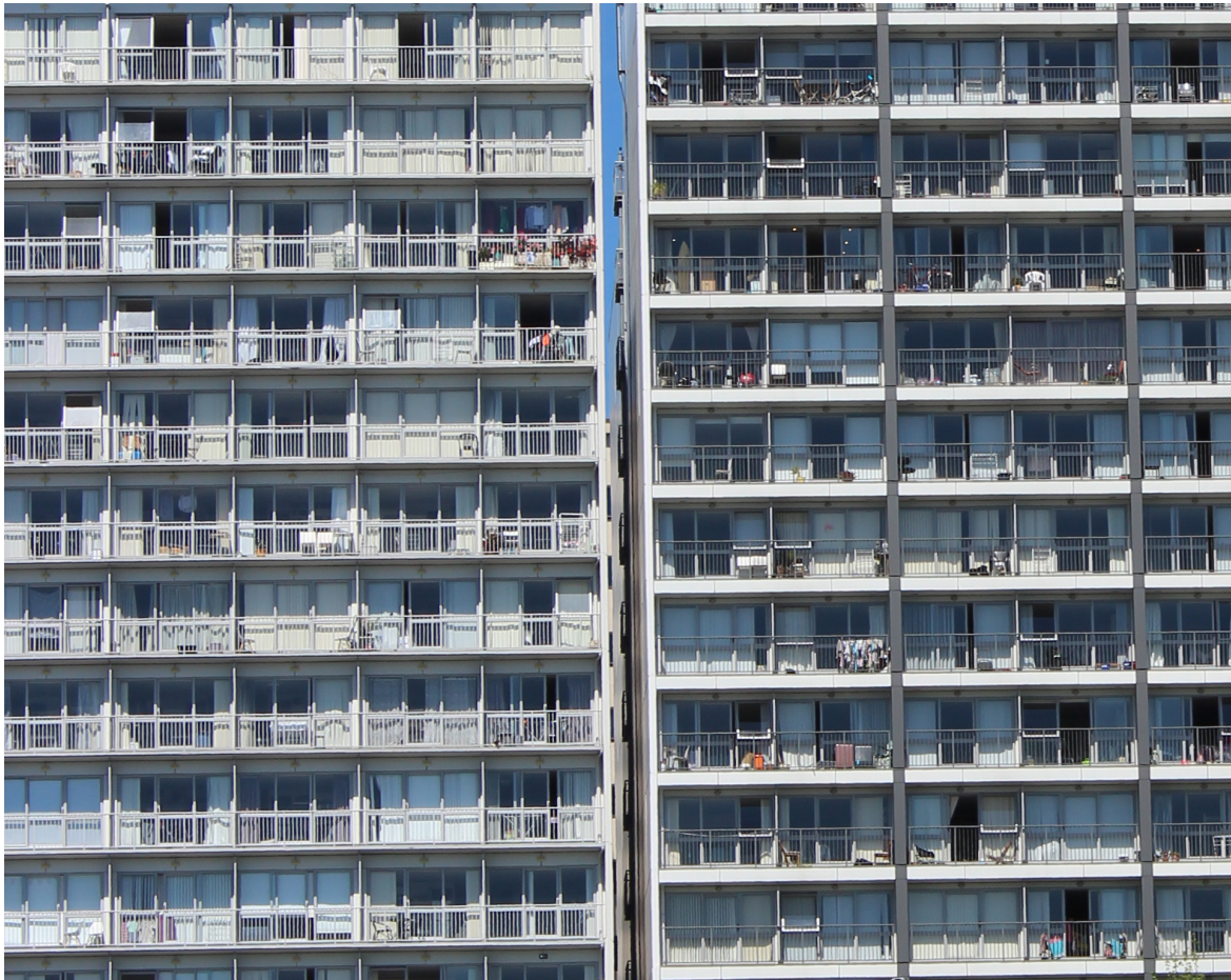
Figure 2.05 - High-Density apartment building in Auckland NZ
