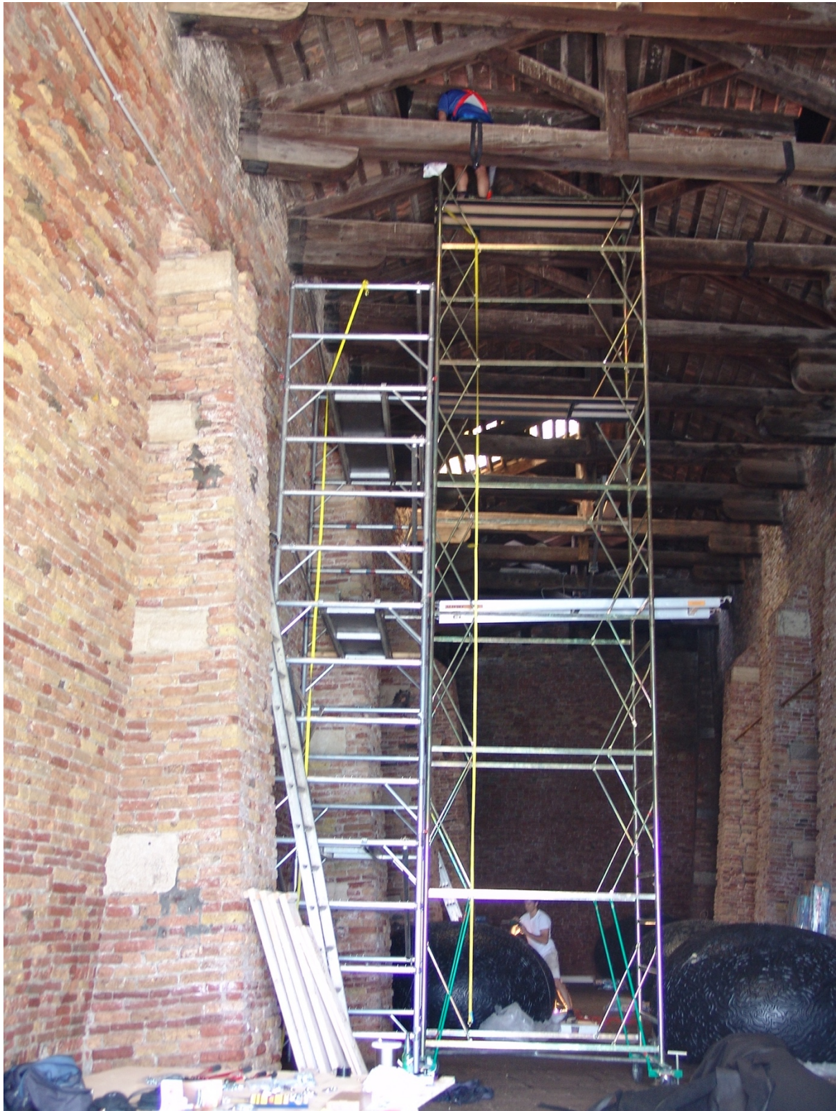
Figure 104: Murray Rich rigs the suspension cables for Āniwaniwa in the heritage-listed wooden rafters of the Magazinni del Sale. Image: Brett Graham Archive.
