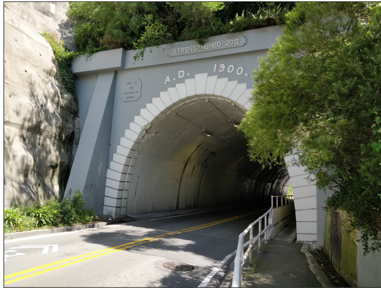
Figure 5.12: Eastern Entrance of the Karori Tunnel. Credit: Author's Own
