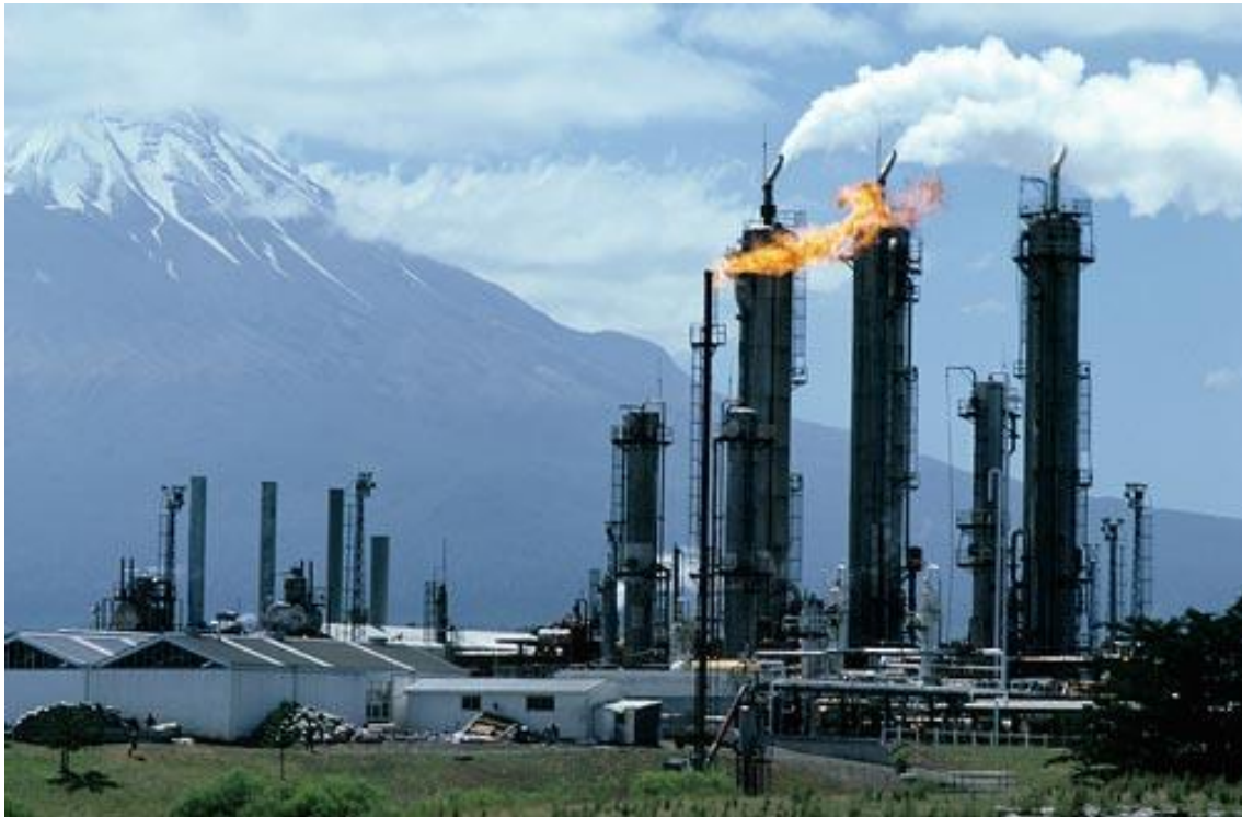
Figure 23: Kapuni CO2 gas extractors
