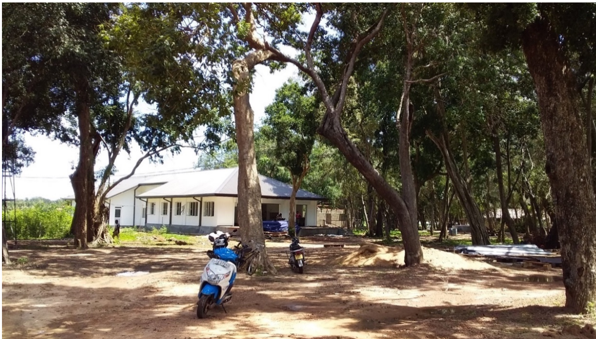
Figure 6.2. Processing plant under construction at the Wannai Dairy Project site.
