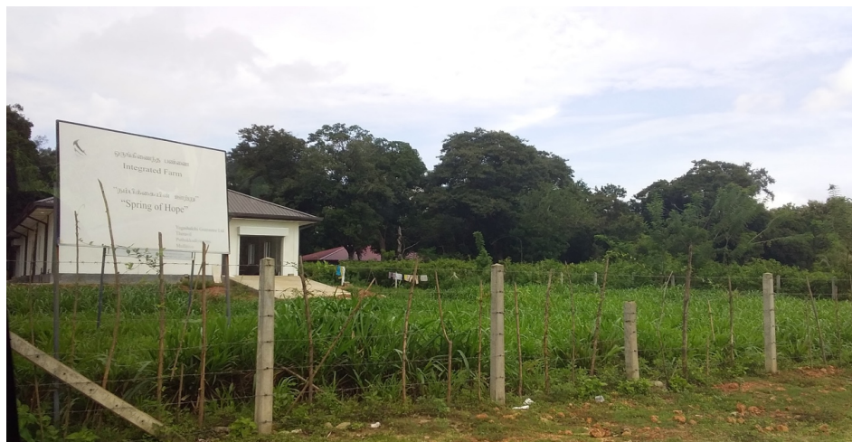
Figure 5.3. Entrance to the model farm, dairy processing plant and project offices.
