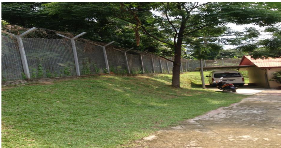
Figure 7: Barbed wire along perimeters of the shelter
