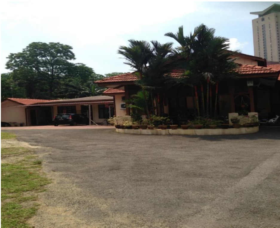
Figure 10: Front view of the shelter building partially hidden by trees
