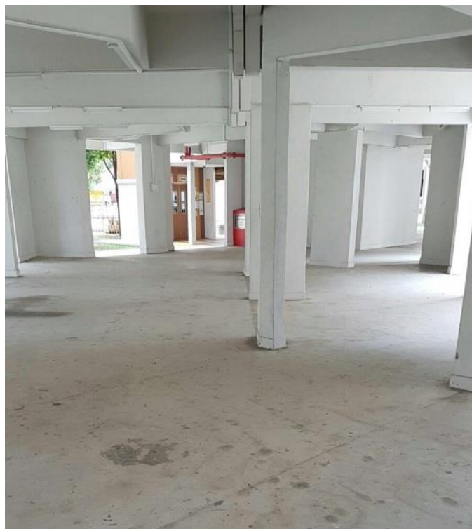
Figure 6.4. Void deck is not void
