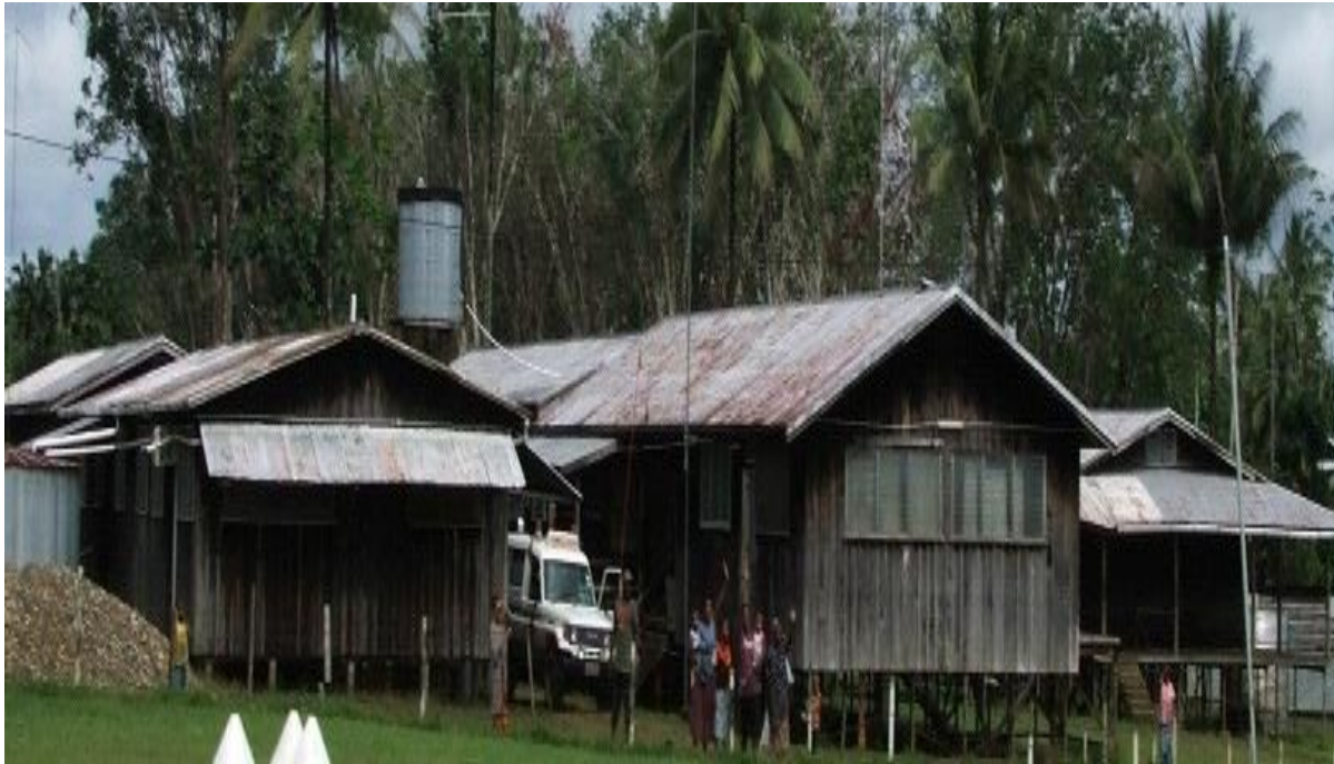
Figure 13. Poor hospital buildings in one of Papua New Guinea rural locations.
