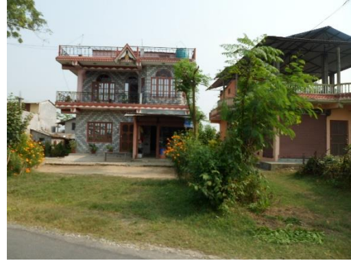
Typical new construction in Chitwan Photo: JJoshi, 2016
