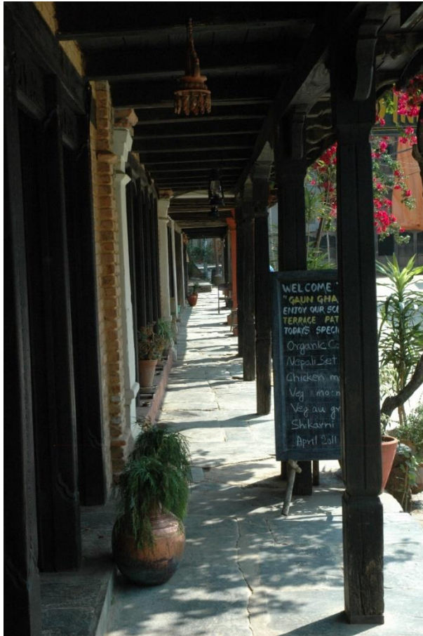
Plate 5-5: Covered passage with balconies on the first level
