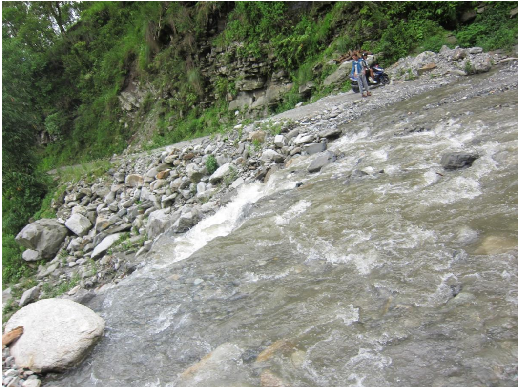
Plate 7-1: Unpaved new road near Kimchi that is flooded in the monsoon seasons
