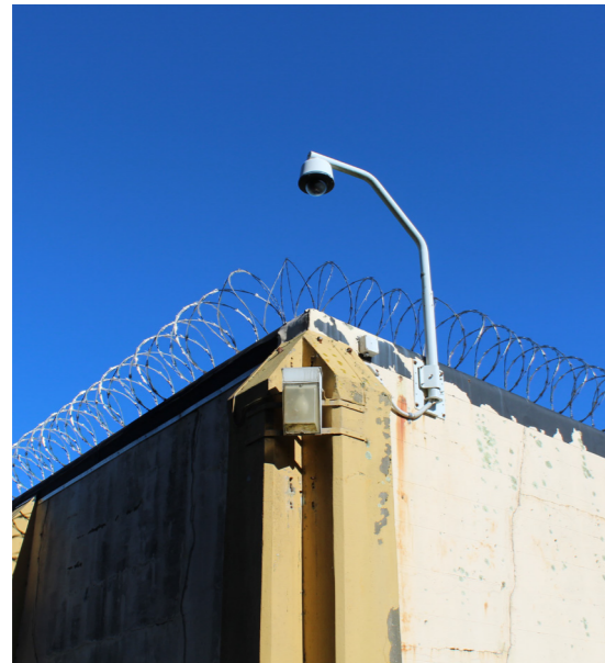
Figure 25. Camera mounted on wall, 2017
