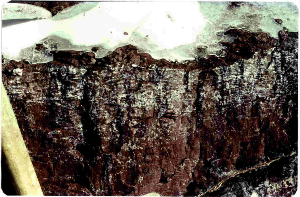
Plate 3.2 Calcite ( \text{CaCO}_3 ) on the vertical surface (type 1A deposit) and in cracks and joints (type 1B) of Aztec Siltstone at Alligator Peak (locality 183). The deposit is thickest immediately below the ledge where snow lies, whereas salt is absent above the ledge. (14/12/73)
