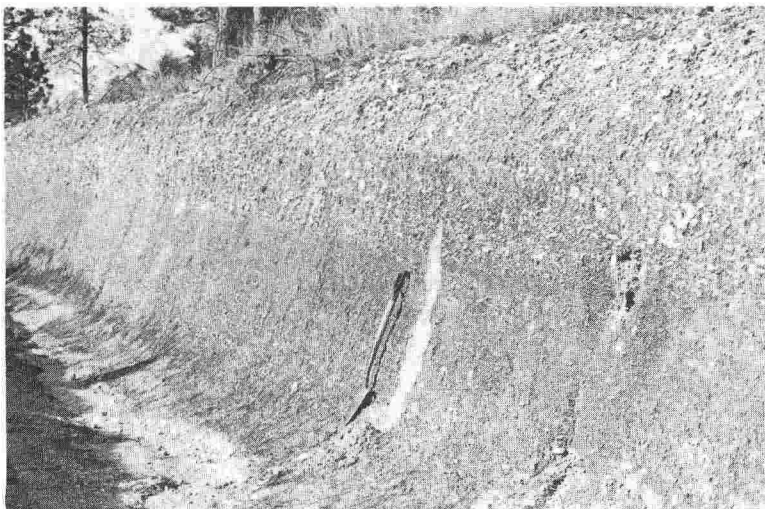
Fig. 11 Section 6, a road cutting through the upper part of Taupo Ignimbrite, beside Rangitaiki River (N94/1862328). Coarse blocky top with sharp lower contact correlates to the Upper unit and is particularly common at the southern part of Kaiangaroa Plateau. Spade 1 m long.
