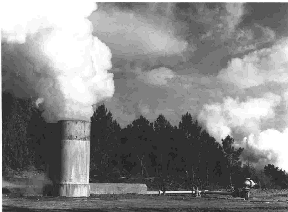
FIG. 8. Bore Br 11 discharging vertically through concrete silencers. Mass output is about 250,000 kg/hour at 10 bars pressure.
