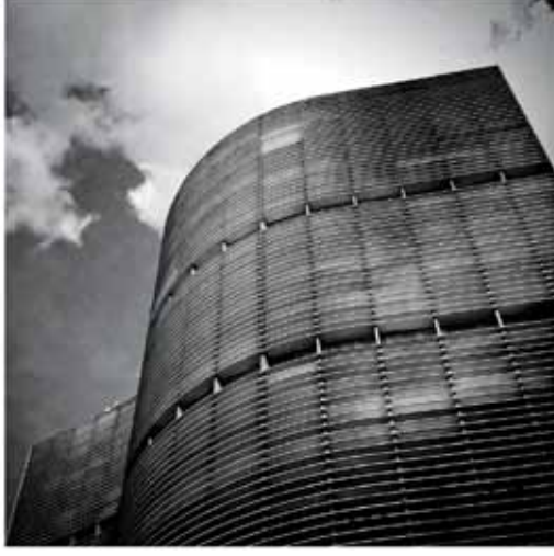
Fig. 37 Copan residential building
