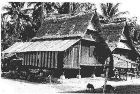
Figure 5-27 A Malay house with an on-stilts system. 35
