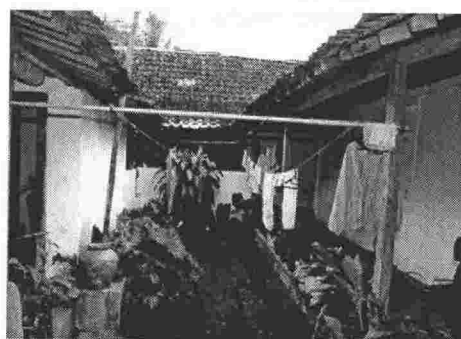
Figure 5-14 A gap between dalem and gandhok .
