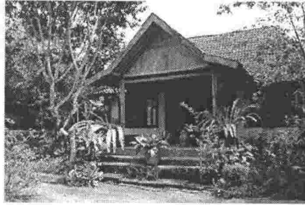
Figure 5-26 A house in Pakem that applies elevated floor system by raising the ground level. Thus, unlike other traditional styles in Indonesia, Javanese buildings do not utilize the space under the floor.
