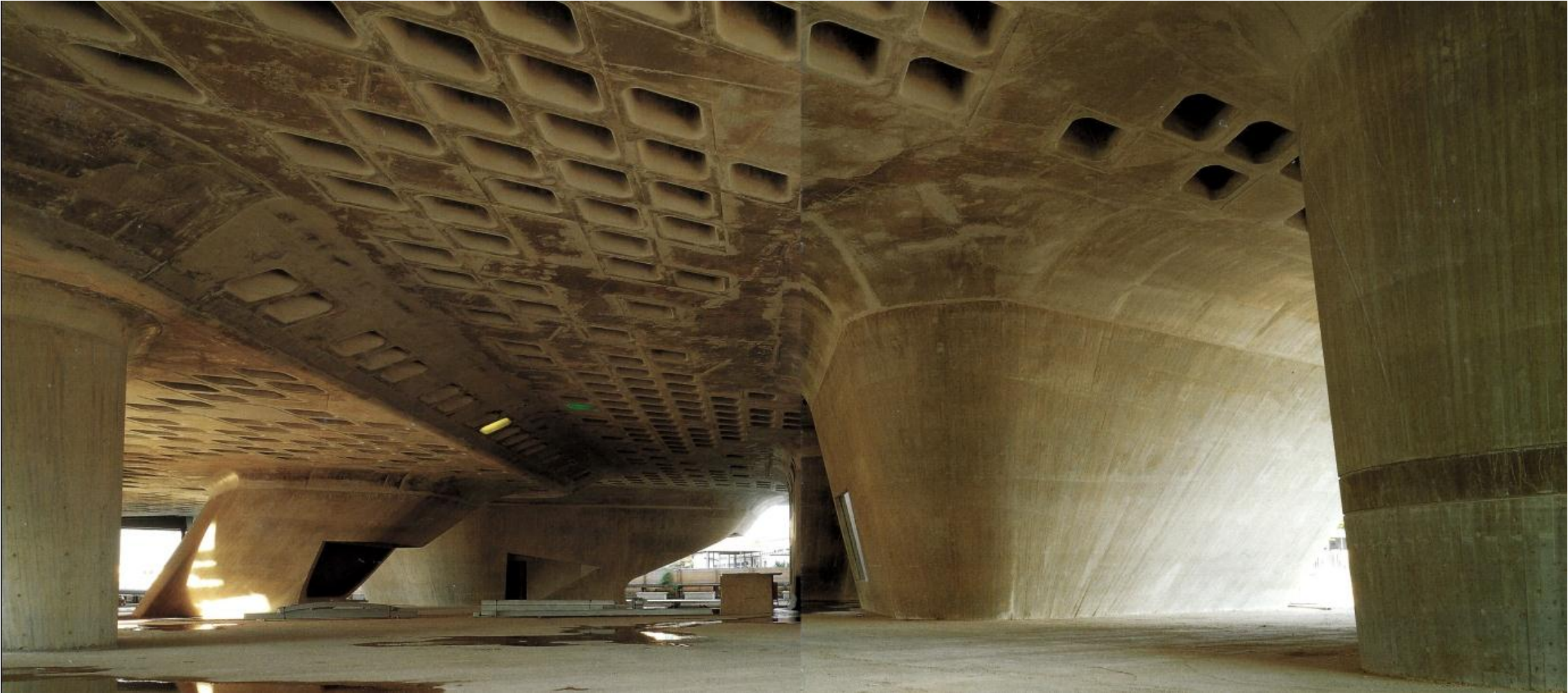
Figure 21: Urban Space during construction located at the ground level of Phaeno
