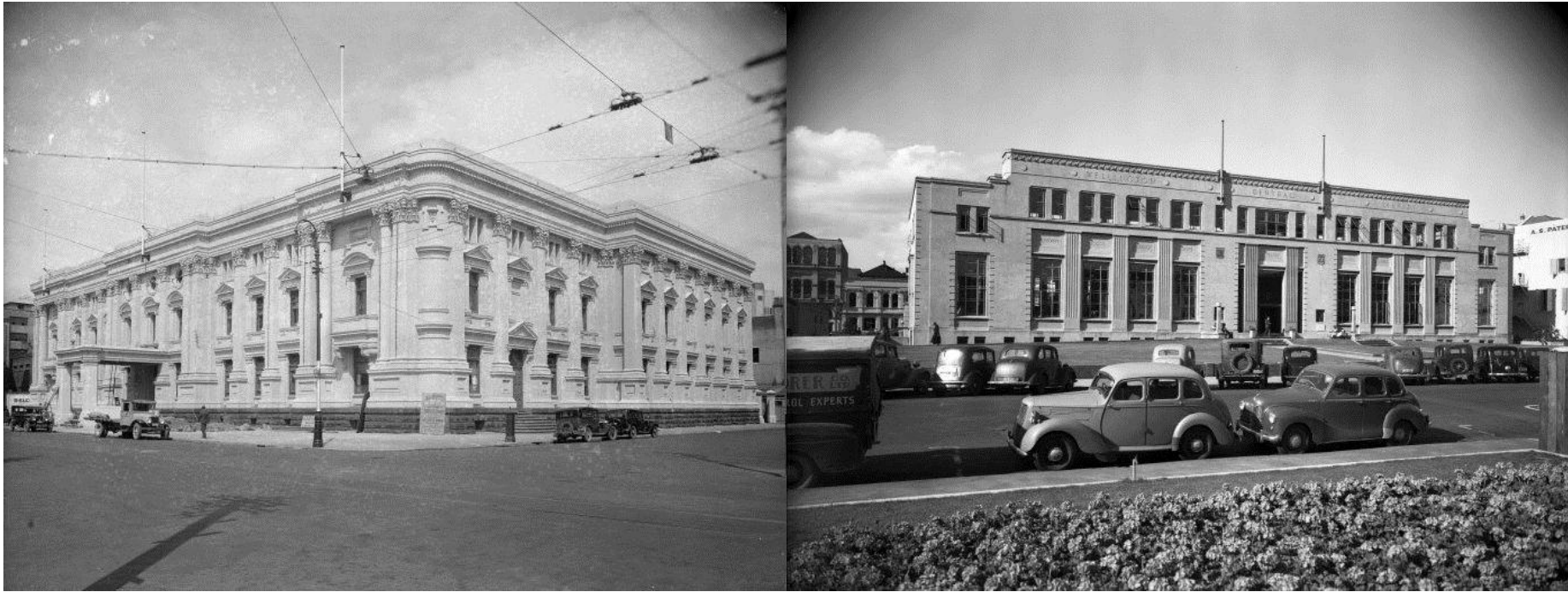
Figure 7-8: On the Left; the Town hall on the corner of Cuba and Mercer Street with its entrance orientated along the now shortened Cuba Street and on the right; opposite the town hall on the Mercer street axis is the original Public Library now the City Gallery. Reference Number: 1/1-015911-F. Photograph taken by Gordon Burt circa 1940.
