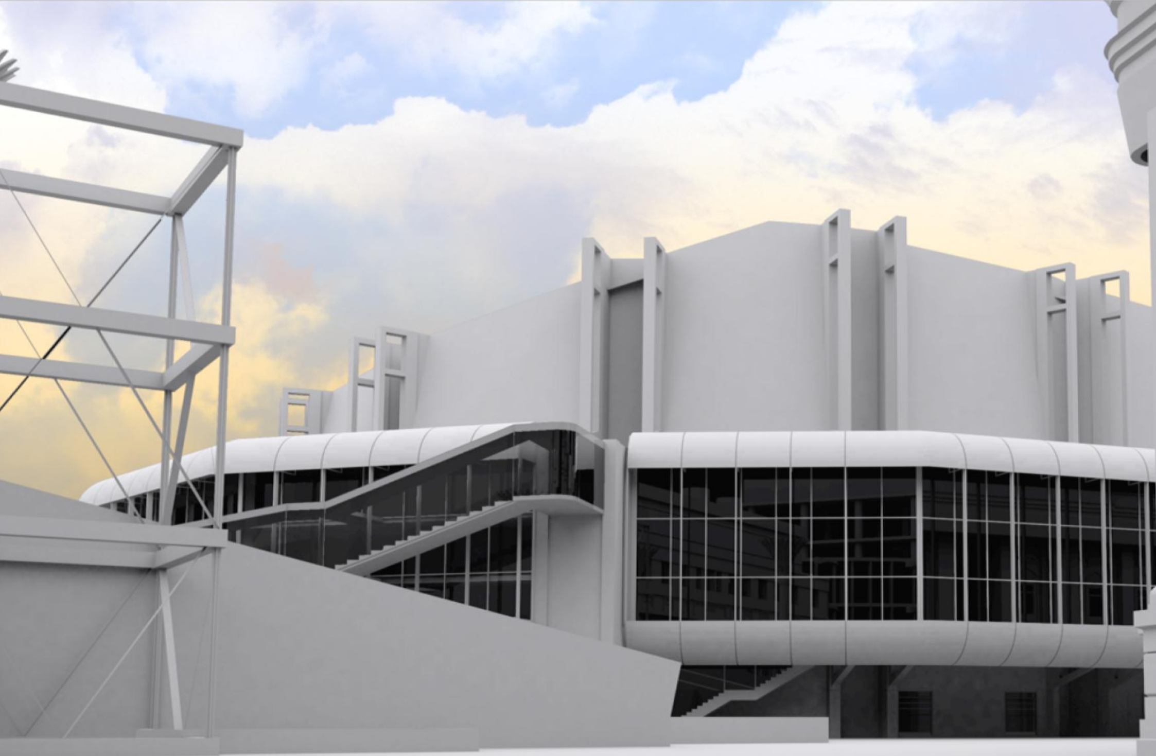
Michael Fowler Centre: object in a field that does not try to resolve the corner of Civic Square, nor does it try to relate to all its grid edges
