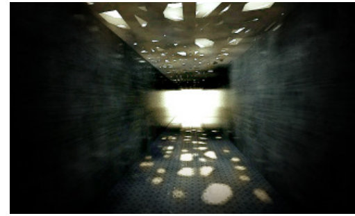
Figure 5.11: Direct light through perforations in corridor
