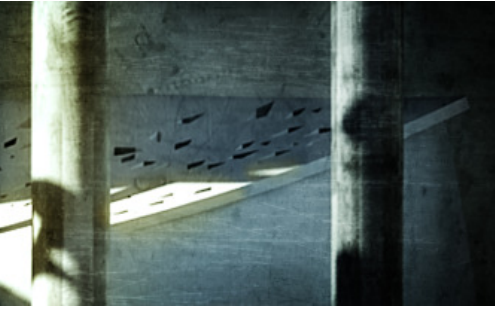
Figure 5.34: Close up of perforated bathroom ceiling
