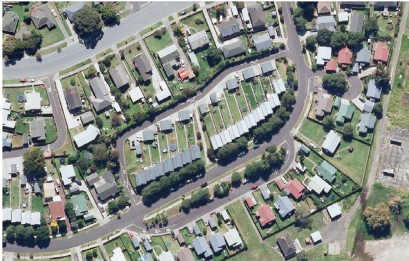
Figure 64. Aerial photograph of part of the Rowena Crescent development. Note its subsidiary roading infrastructure and how pedestrian connectivity is increased by central lot-wide lanes.
