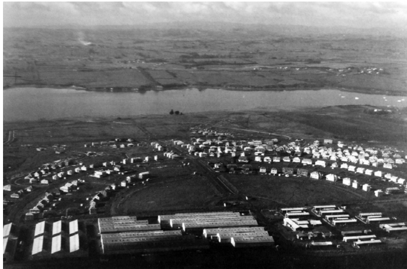
Figure 31. Aerial view of the southern end of the Tamaki state housing scheme, (Northern Panmure). Its concentric crescents reflect Garden City planning principles (Archives New Zealand - AALF 6112/3, 18/2/15).
