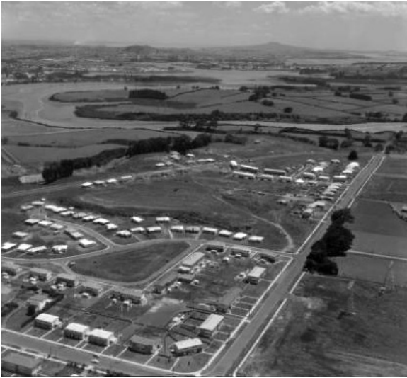
Figure 79. A 1961 aerial photograph of part of the Otara design case study area. Ngati Otara Park and the Tamaki River can be seen in the distance (Alexander Turnbull Library - WA-56602-F).
