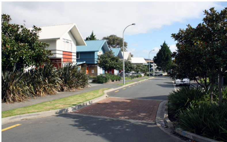
Figure 16. Part of the Talbot Park Community Renewal project that replaced earlier duplexes with a variety of housing types. Author's own image.
