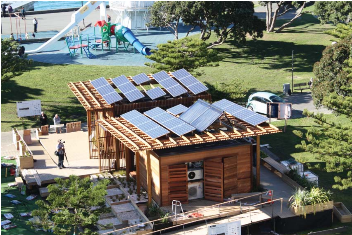
Figure 82: First Light house on Frank Kitts park from above
