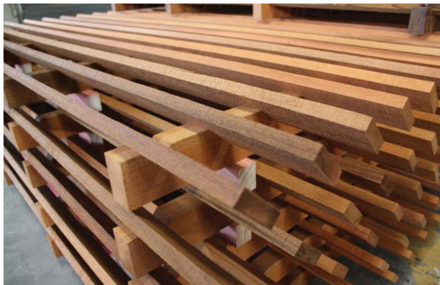
Figure 51: Canopy slats stacked during construction
