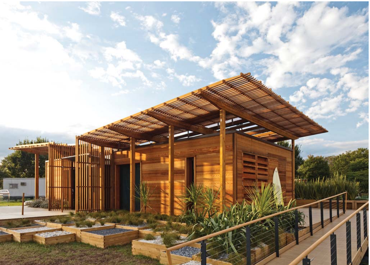
Figure 1: Image of completed house in Washington DC
