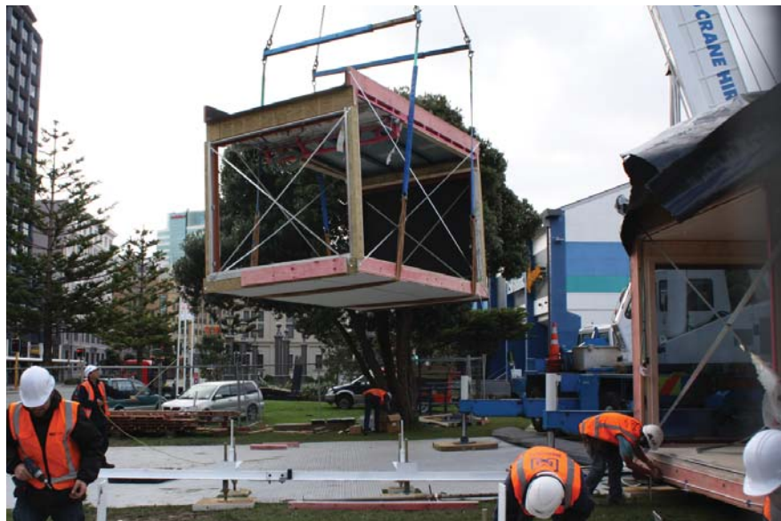
Figure 28: Craning the modules into place on Frank Kitts Park
