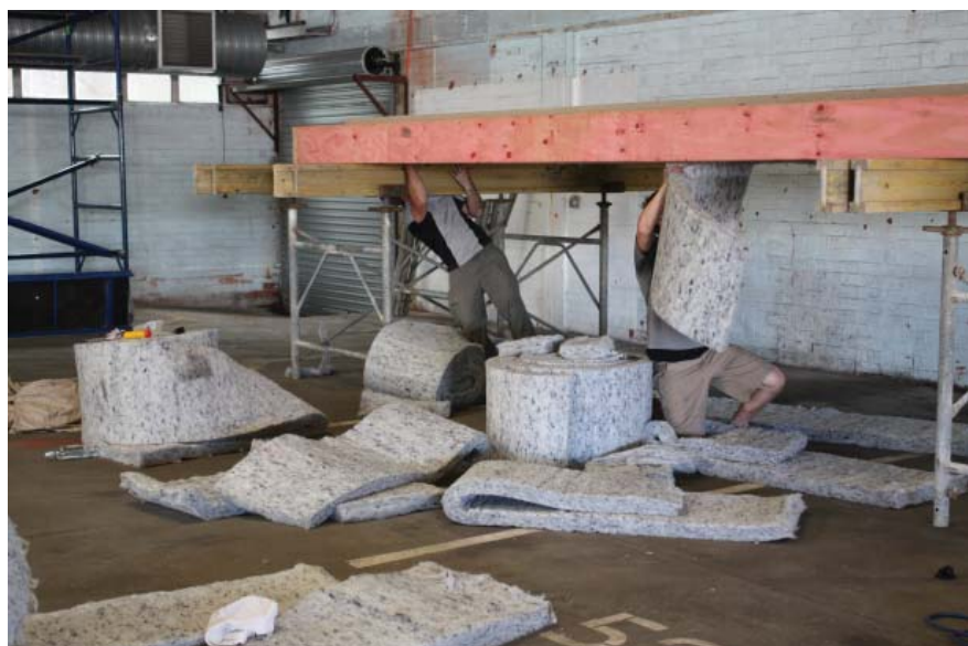
Figure 21: Installation of wool insulation
