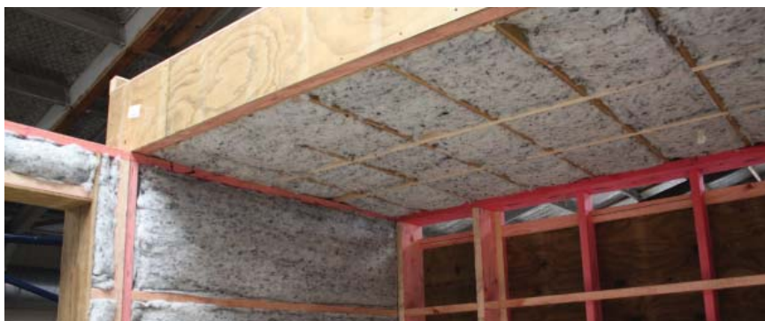
Figure 22: Installed wool insulation in roof and wall
