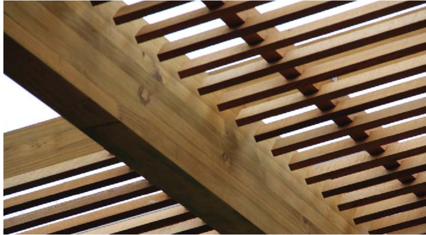
Figure 52: Angle of installed canopy slats
