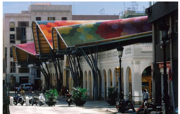
Figure 28. Santa Caterina Market, new canopy draped over old facade.
