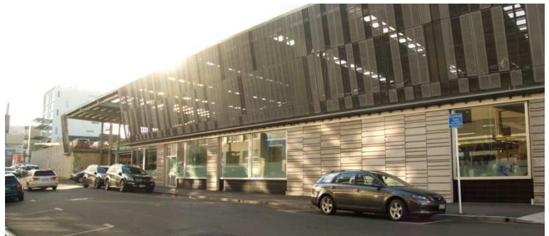
Figure 22. Moore Wilson's, College Street looking towards Tory Street.
