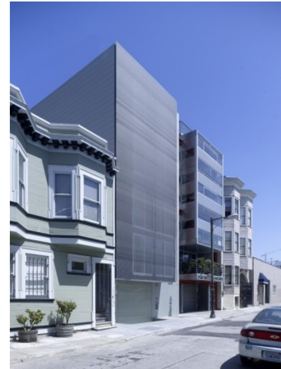
Figure 1.8 - 1028 Natoma Street, San Francisco, Stanley Saitowitz - an example of rejecting the context - the Victorian townhouse form is ignored and an unsympathetic modern block is inserted
