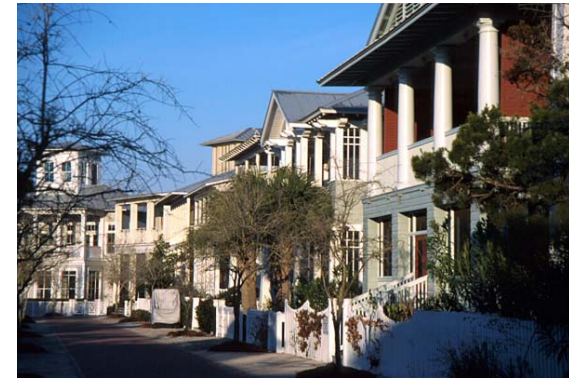
Figure 1.6 – Houses in Seaside, Florida - this New Urbanist development replicates traditional house forms
