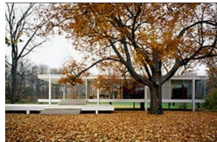
Figure 5.7 : Farnsworth House entrance
