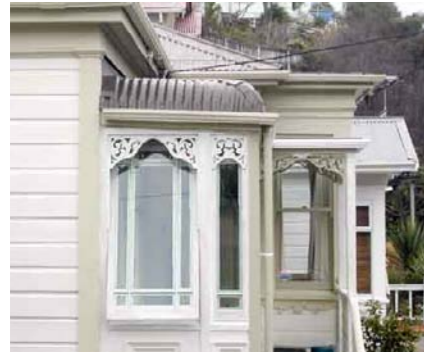
Figure 4.1: Restored Kilbirnie villas, Wellington
