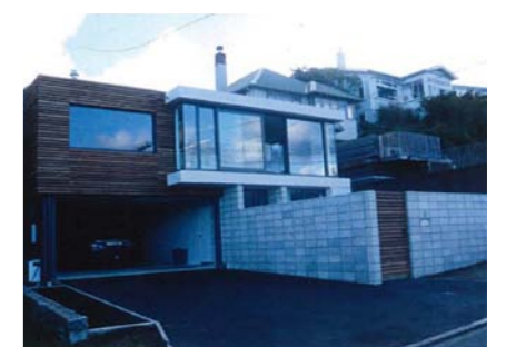
Figure 6.6: Street elevation after latest alterations
