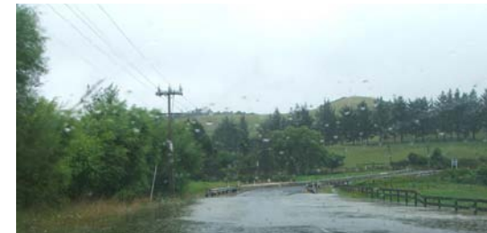
Figure 89. Flooding on the main Matarangi access road.
