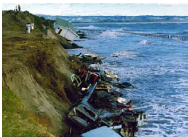
Figure 12. Severe erosion at Ohiwa Spit, Waikato
