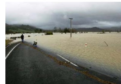
Figure 65. Flooded access road, Pauanui.
