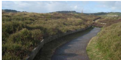
Figure 46. Public walkways through dunes at southern end of spit
