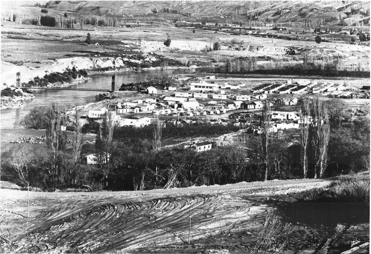
C2: A view of the camp at the hydro-electric works at Roxburgh gorge. The south end of the deviation is seen in the foreground and the Bailey bridge spanning the Molyneux is to the left, 21 September 1949 (Photographer: Jack Debnam Stewart Roberts. NZ Free Lance Collection, Alexander Turnbull Library, Wellington, NZ. Ref#: C-1746-1/2)
