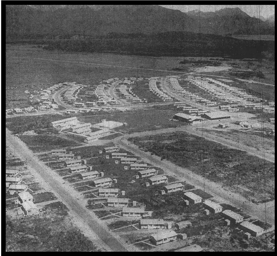
Figure 20: Manapouri construction village
