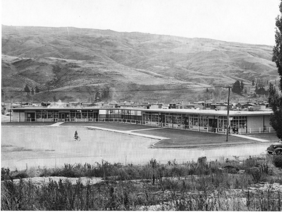
C5: Shopping centre at the Hydro Electric Station, Roxburgh, June 1952 (NZ Free Lance Collection, Alexander Turnbull Library, Wellington, NZ. Ref #: F-45713-1/2)
