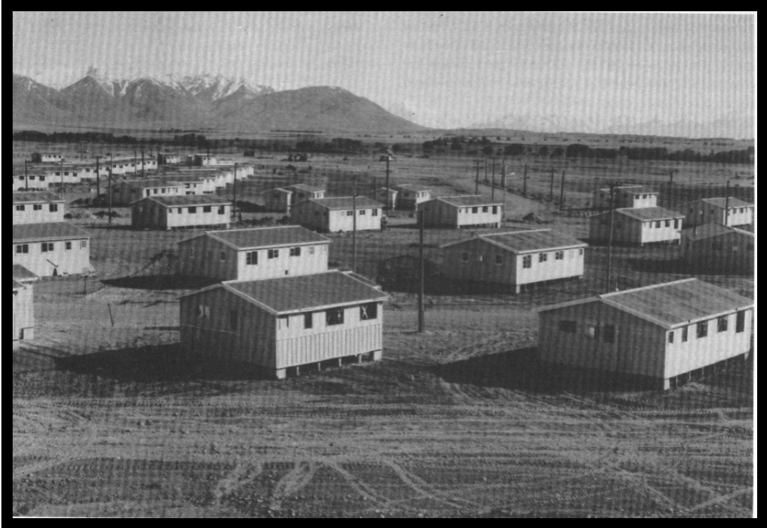
Figure 23: Houses in place at Twizel
