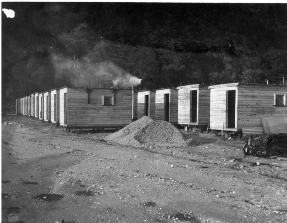
E6: Huts placed on foundations at West Arm (Photo by Ministry of Works and Development, courtesy of Meridian Energy)
