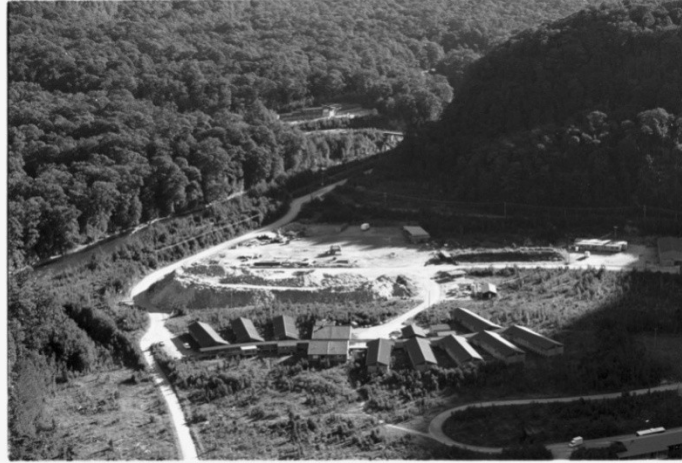
Figure 2: 2MTT construction camp, 1999
