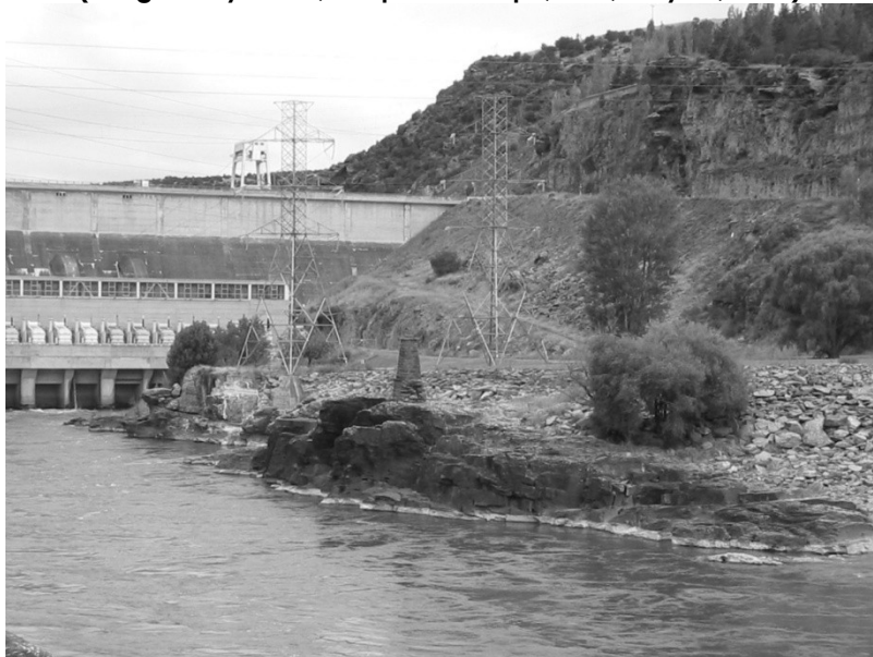
C8: Roxburgh hydro village site 2005 (Photo by the author)
