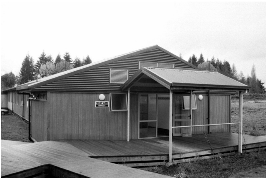
H13: 2MTT hostel sections in place at Te Anau Holiday Park, 2004 (Photo by the author)
