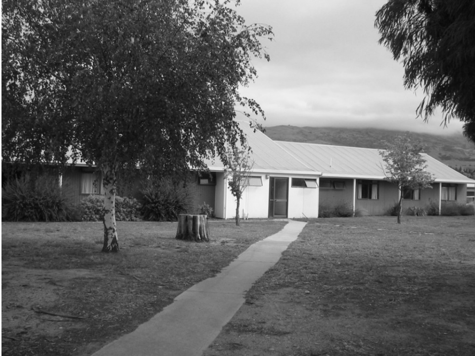
G8: A section of the Zublins' staff hostel, in use at Cromwell Holiday Park, 2007 (Photo by the author)
