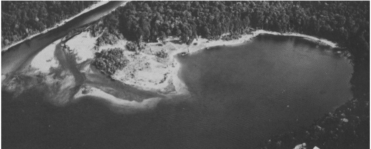
E2: West Arm prior to the beginning of 1MTT construction (Photo by Ministry of Works and Development, courtesy of Meridian Energy)
