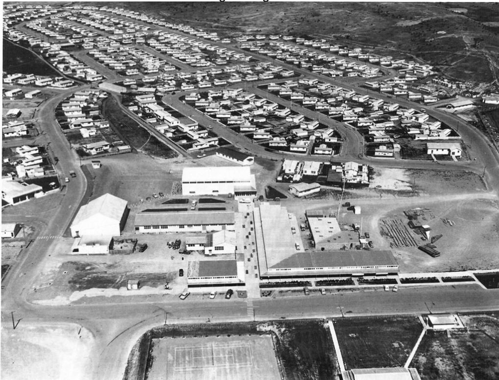
D3: Ministry of Works township of Otematata, 1960 (Alexander Turnbull Library, Wellington, NZ. Ref #: PICT-000085)
