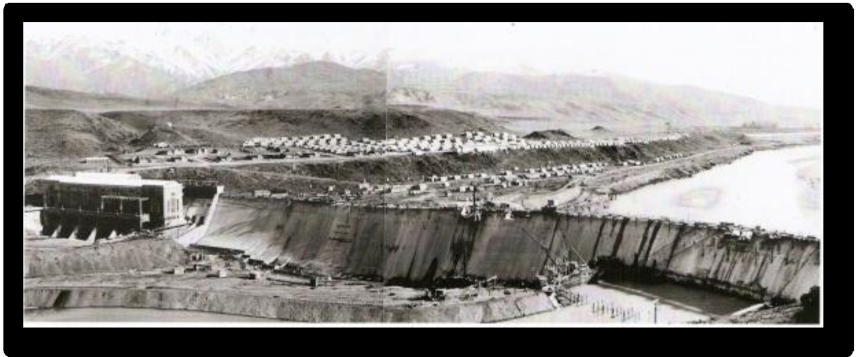
Figure 7: Waitaki Hydro electric station and construction camp, August 1934
