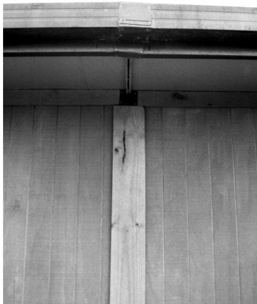
H12: 2MTT hostel sections joined at Te Anau Holiday Park (Photo by the author)
