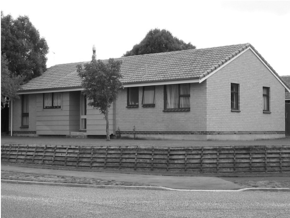
G6: Masonry clad hydro project house at Cromwell, 2007 (Photo by the author)
