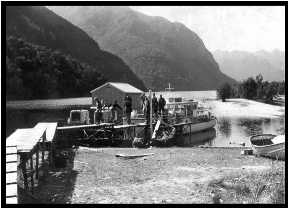
Figure 13: The first hut being delivered to West Arm, 1963
