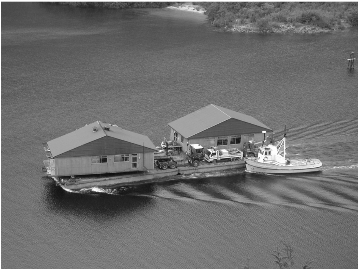
H9: 2MTT hostel sections being barged out of West Arm (Photo courtesy of Meridian Energy)
