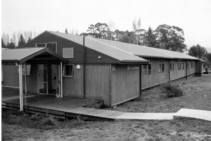
H14: 2MTT hostel sections in place at Te Anau Holiday Park, 2004 (Photo by the author)
