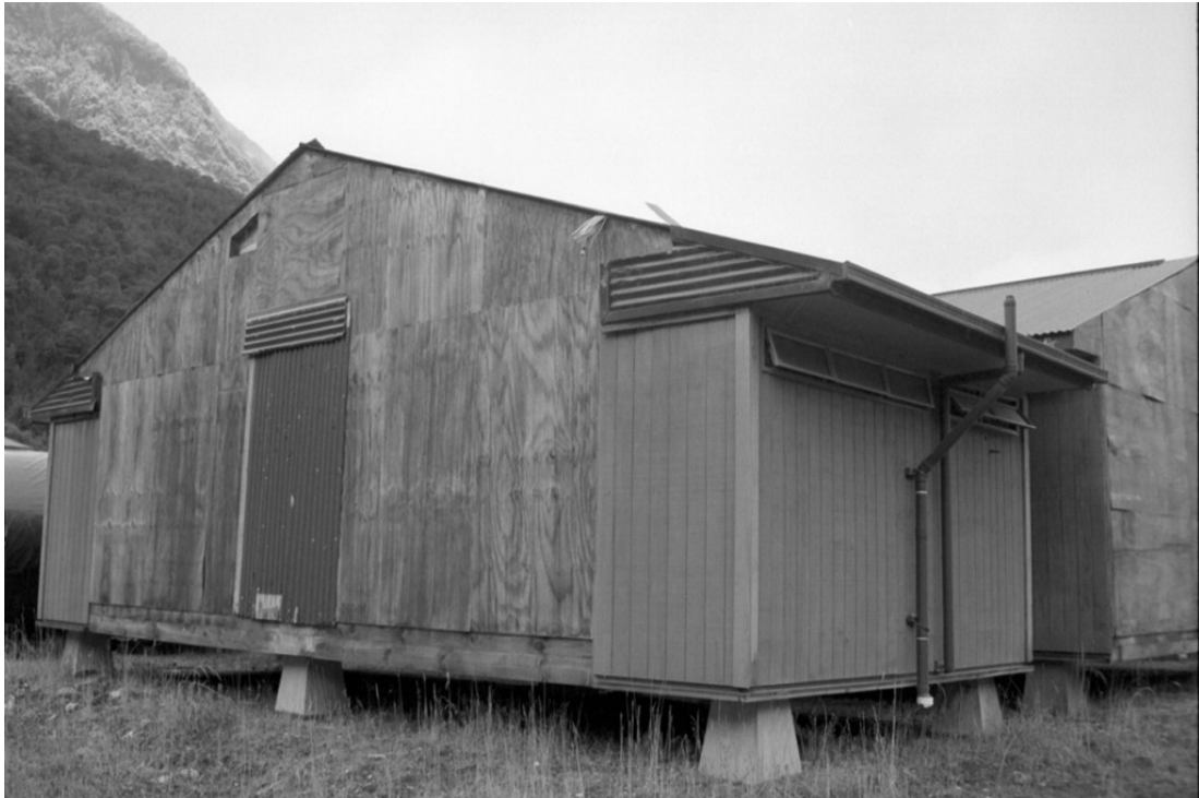
H6: 2MTT hostel section at West Arm awaiting transportation off site, 2004 (Photo by the author)
