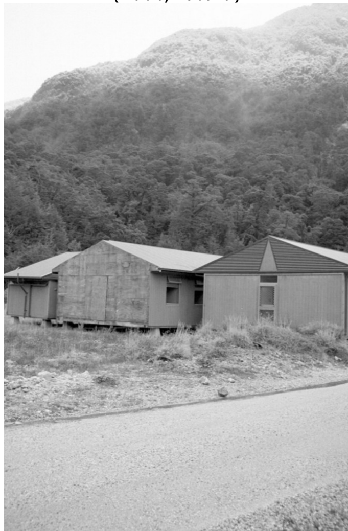
H5: 2MTT hostel section at West Arm awaiting transportation off site, 2004 (Photo by the author)
