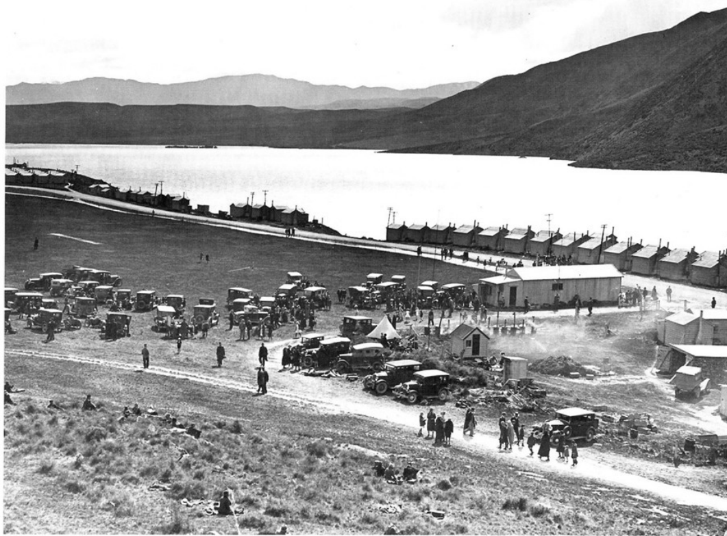
B3: Visitors at Waitaki Hydro dam on picnic day, 4 October 1934
