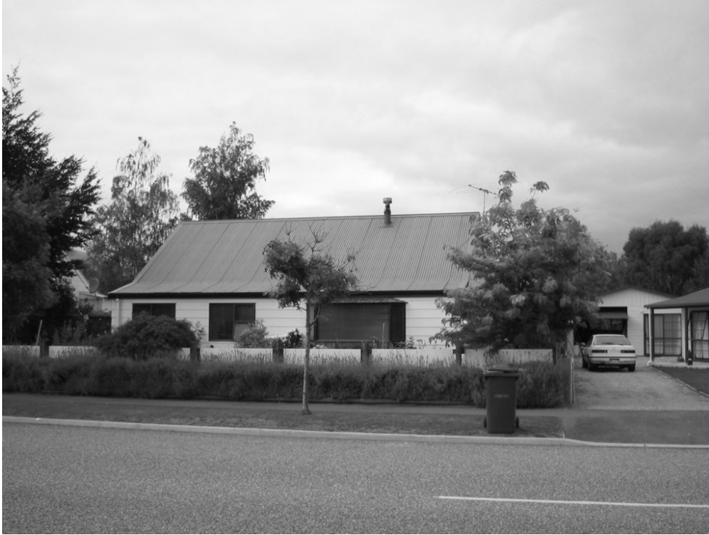
G4: Lightly clad hydro project house at Cromwell, 2007 (Photo by the author)
