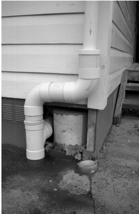
E13: 1MTT hostel relocated to Te Anau Holiday Park (Photo by the author)
