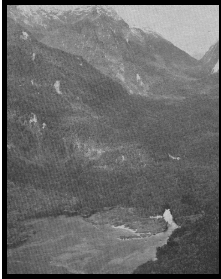
Figure 30: Deep Cove prior to the beginning of construction (Photo by the Ministry of Works)
