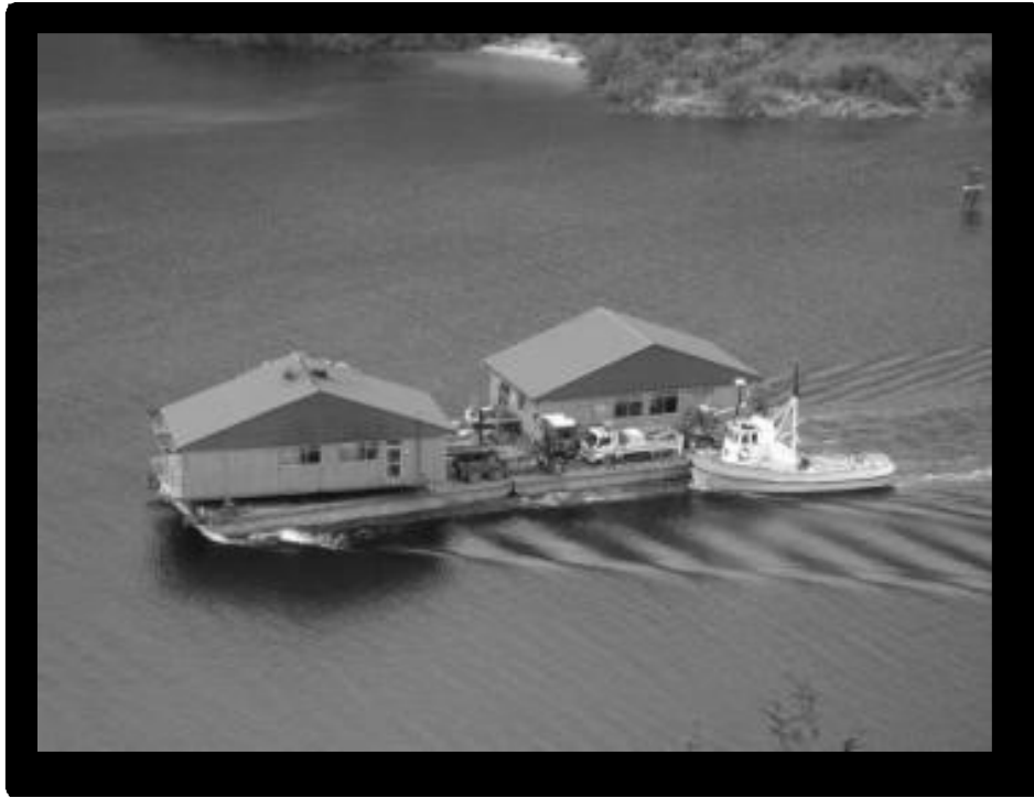
Figure 26: West Arm FDI staff hostel sections being barged out, 2002
