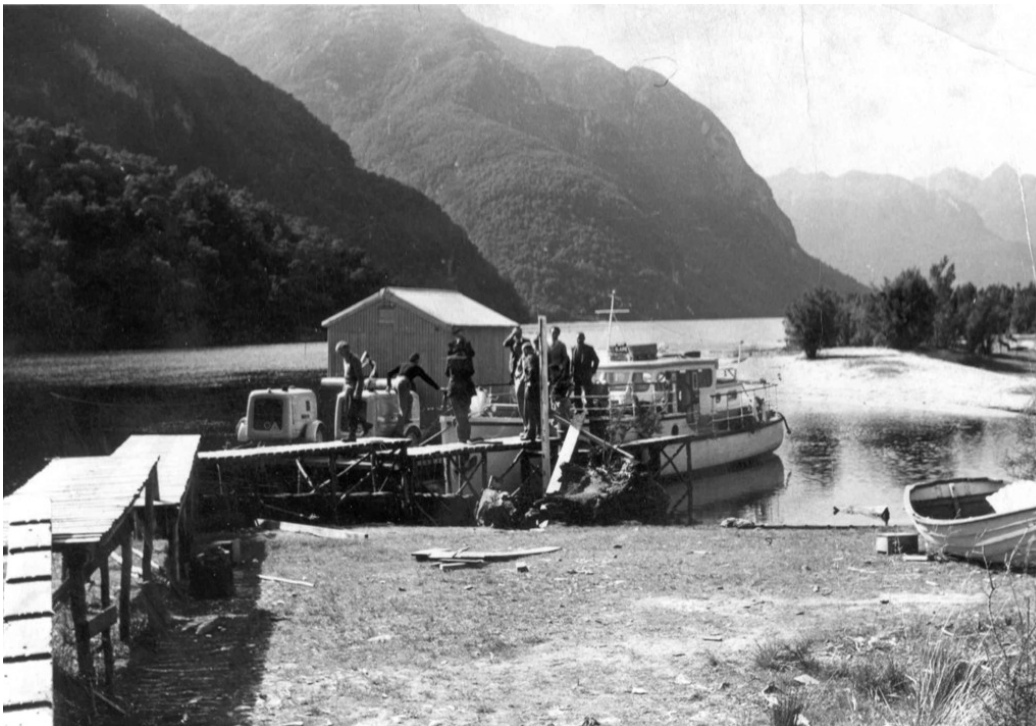
E21: 1MTT Deep Cove Shore Camp hut being barged in (Photo by Ministry of Works and Development, courtesy of Meridian Energy)
