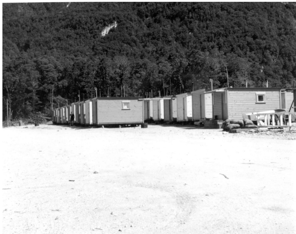
E7: 1MTT huts at West Arm (Photo by Ministry of Works and Development, courtesy of Meridian Energy)
