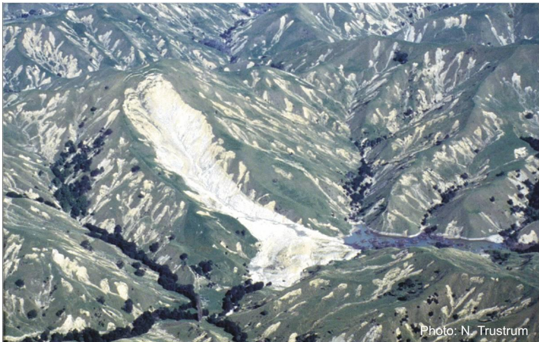
Figure 3.31. Storm induced slope failure. Shallow and deep-seated landsliding at the Mangakiore field site following the Bola event 1988 (Photo Trustrum 1988).
