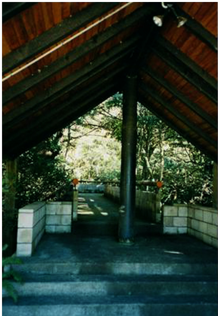
Figure 17. Aniwaniwa Visitors Centre elevated walkway, Under the shelter of the Waharoa. Image by Author, 2003.
