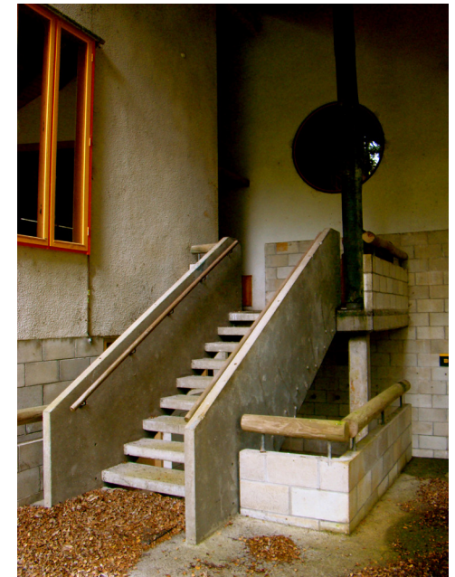
Figure 24. Approaching the building # 4. Image by Author, 2010.
