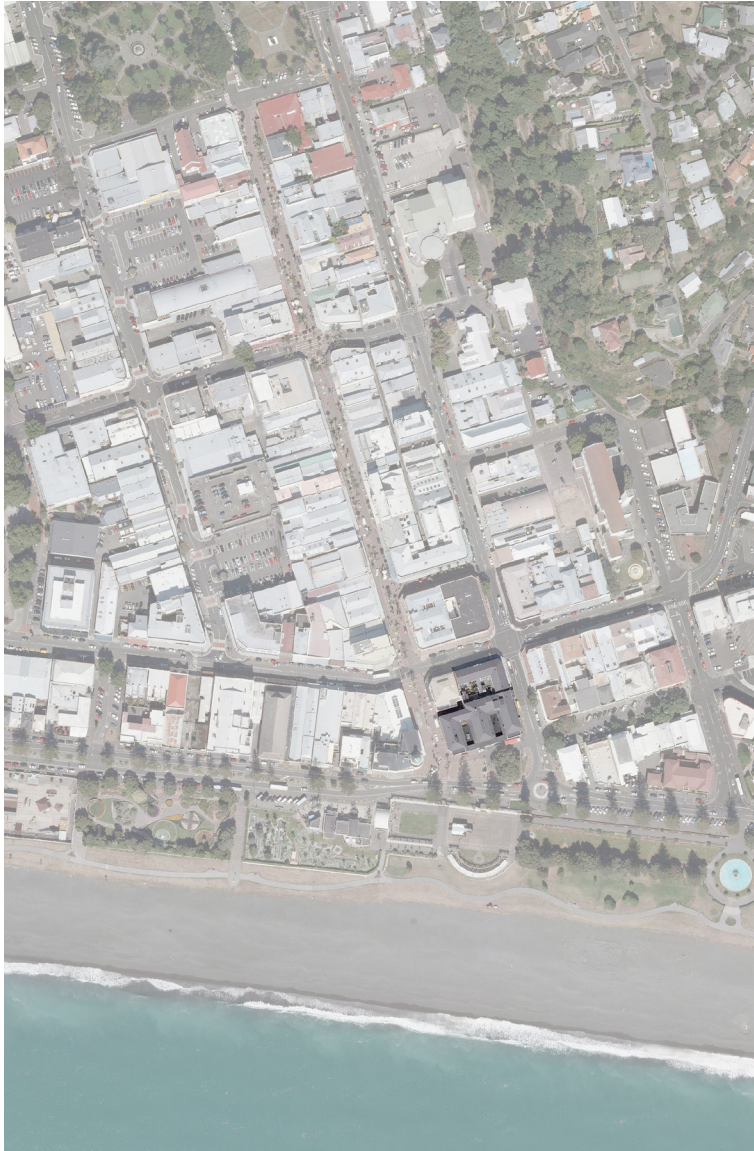
Figure 46. Aerial view of The Masonic in the wider context of Napier City. Image sourced from The Napier City Council, 2010.
