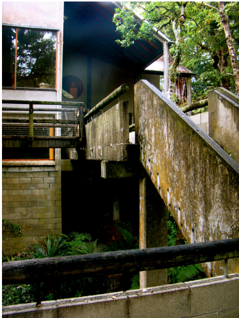
Figure 21. Approaching the building. Image by Author, 2010.
