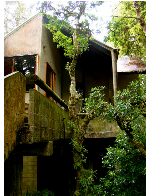
Figure 23. Approaching the building # 3. Image by Author, 2010.
