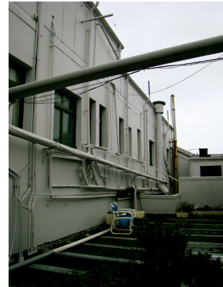
Figure 42. View of open courtyard in the Hastings Street end wing. First Floor. Image by Author. 2010.
