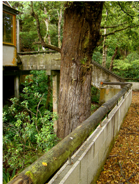
Figure 18. Aniwaniwa Visitors Centre elevated walkway, Beyond the Waharoa and into the bush. Image by Author, 2010.
