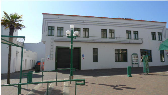
Figure 36. The Masonic Hotel Emerson Street Elevation. Image by Author. 2010.
