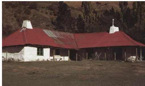
Figure 25: Esk Head Homestead, 1863 in North Canterbury
