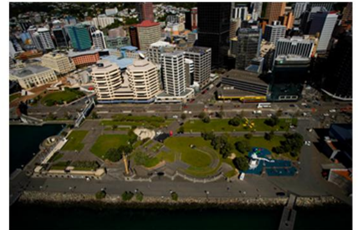
15. Total Site Aerial View
