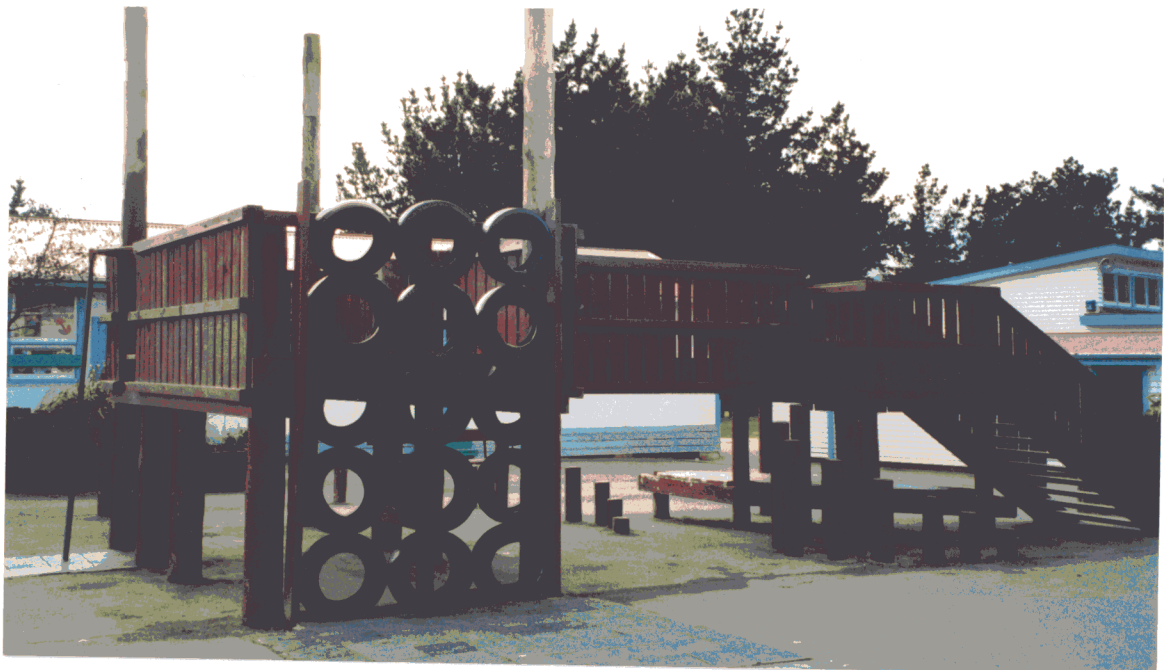
Fig 17 Play ground climbing equipment With safety matting below
