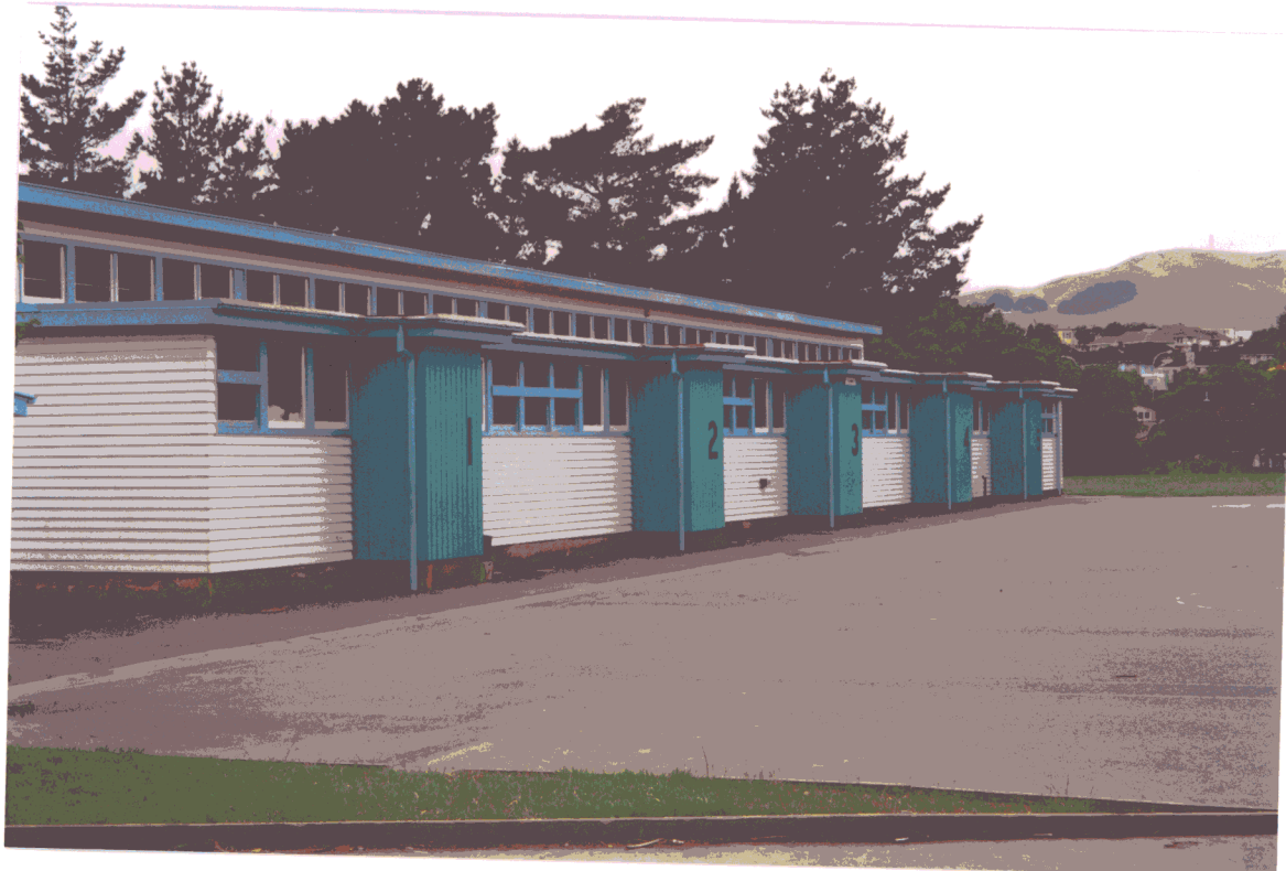
Fig 19 Cannons Creek School classroom block 3
