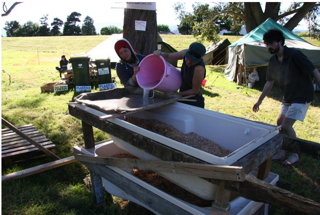
Figure 4.9. 'Doing it ourselves' sustainability: Participants emptying waste water into the grey water system (Source: John Darroch)
