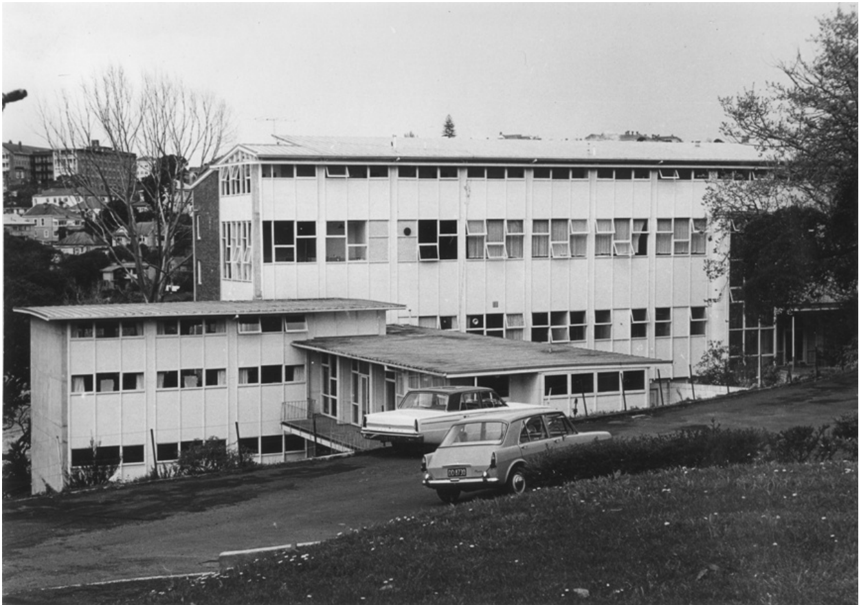
Figure 6. Administration wing (right) and Library (left) at Whitaker Place (1968)
