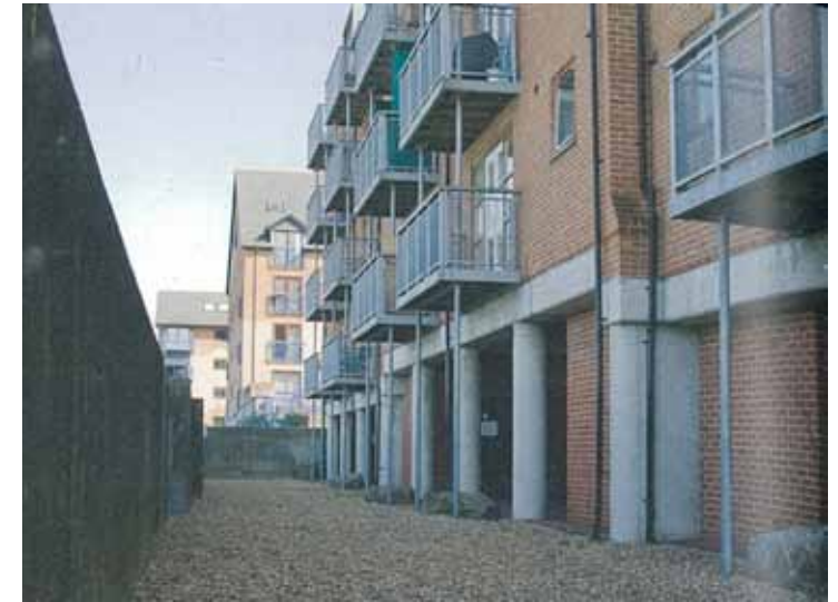
Fig 4.4 Sea Wall in Northampton, Britain Flood defences can create unwelcoming public spaces
