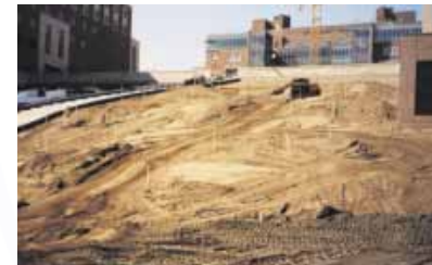
University of Minnesota Minneapolis, Minnesota Riverbend Commons, at the University of Minnesota, reclaimed its view of the Mississippi River by replacing an above-ground parking ramp with an underground structure. Concerned over the stress that landscape soils would impose on the structure, engineers significantly reduced structural loads by specifying geofoam to create their landscape.
