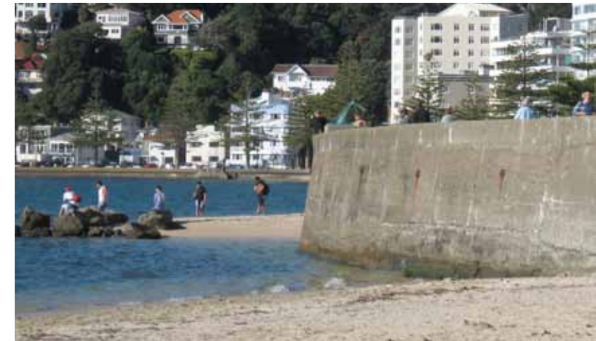
Fig 4.15 An existing sea wall at Oriental Bay, Wellington
