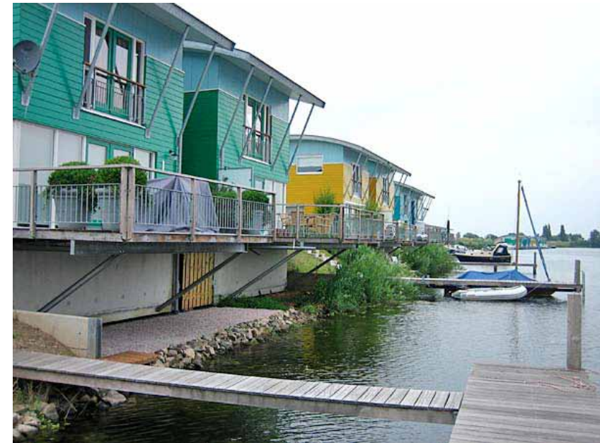
Fig 4.5 Amphibious houses, Maasbommel, Netherlands These buildings sit on dry land by the lakeside. Others further down the shore sit on piles in the lake itself.
