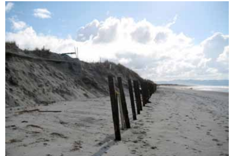
Fig 2.2 Coastal erosion of Waihi Beach, Coromandel Peninsula, NZ Wave action threatens coastal protection structures.
