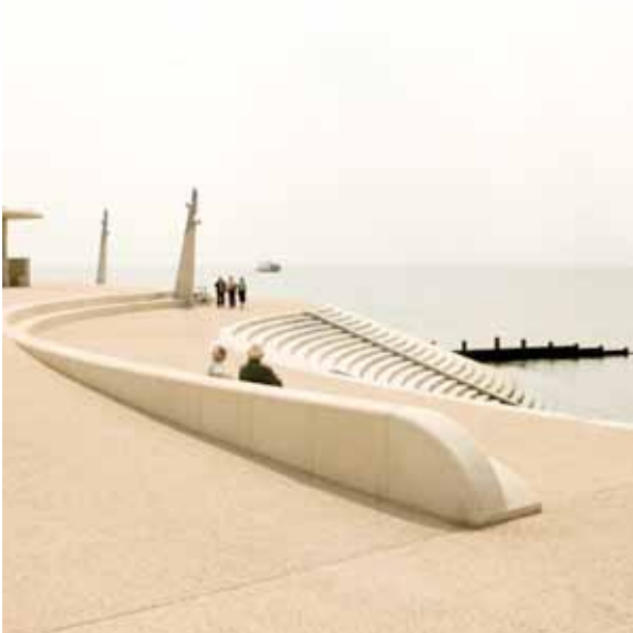
Protect Cleveleys Seawall, Lancashire
