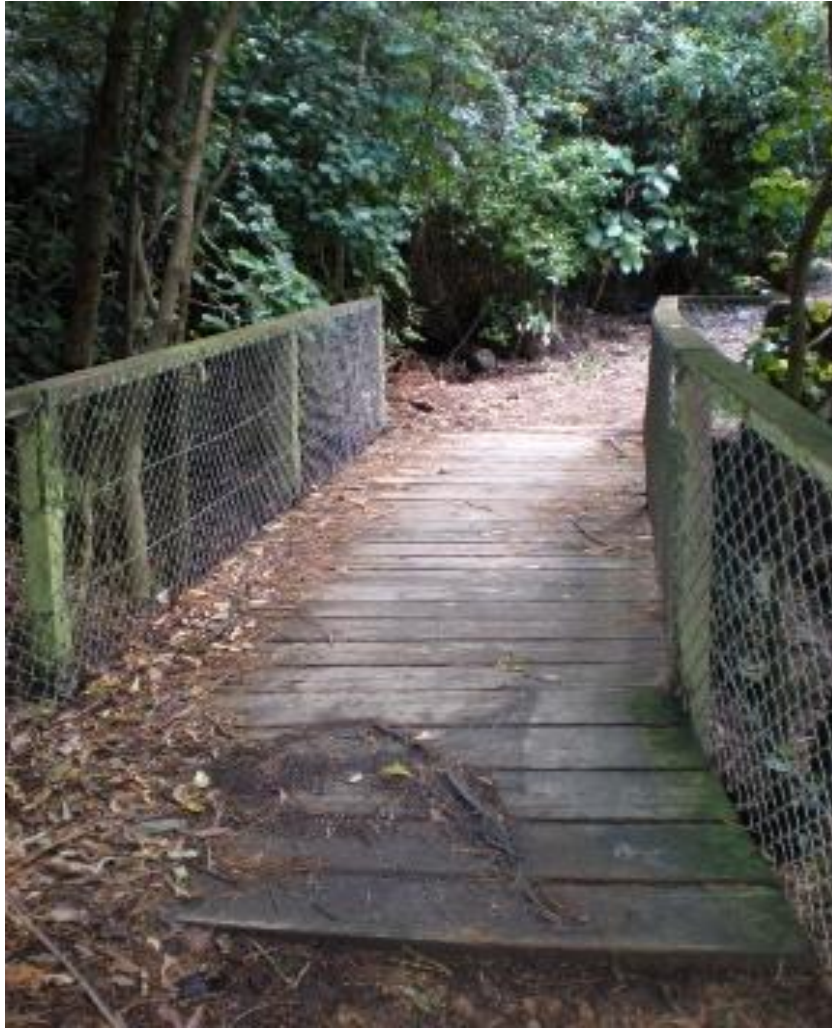
Photo 6: Bridge in Central Park
