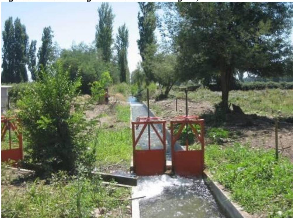
Figure 6.7. Arterial irrigation canal and control gates, Yerbas Buenas
