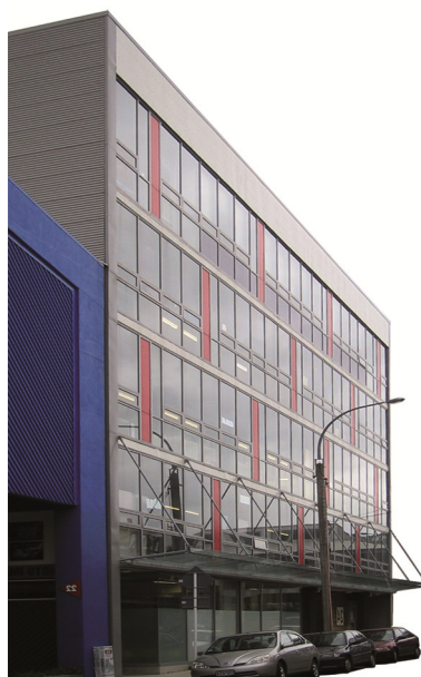
Figure 3:1: Wigan Building facing Wigan St, taken by the author on May 2009
