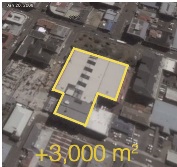
Figure 7:22: Aerial View of SoAD roof space 200
