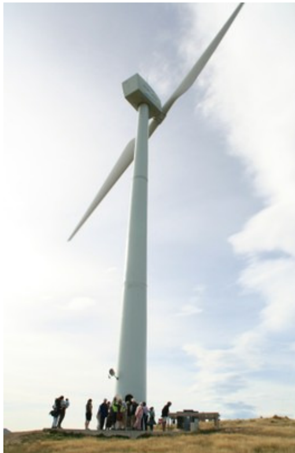
Figure 7:24: Photo of Windflow 500 with the two-blades spanning 33m
