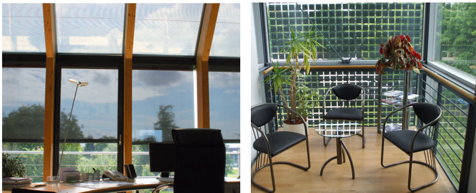
Figure 62: Amorphous silicon thin film cells and microcrystalline silicon bottom cells integrated in glazing
