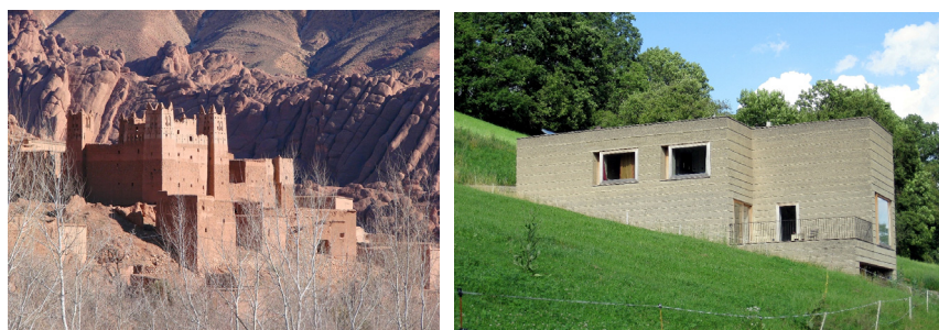
Figure 37: Traditional clay building (Kasbah in Morocco) and modern clay house in Austria
