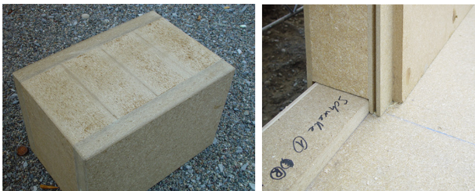
Figure 42: Sample of a Stropoly panel and a door sill and wall detail on the site
