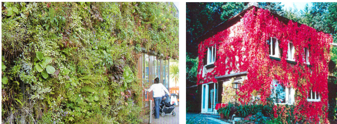
Figure 48: Hydroponics green wall system with over 170 plant species and a house covered with Virginia creeper
