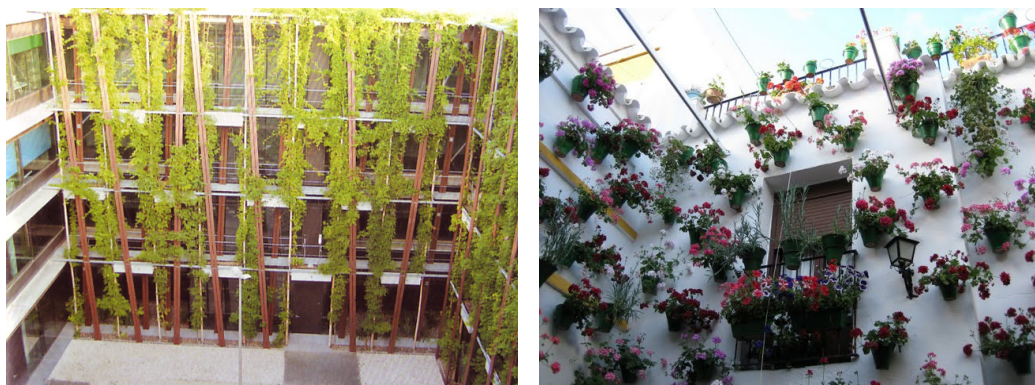
Figure 46: Shading provided by climbing plants and traditional patio in Cordoba, Spain
