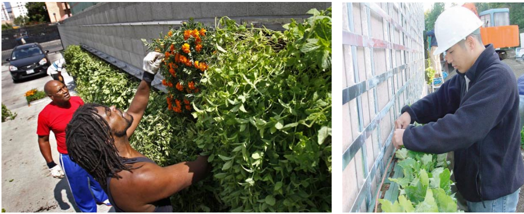
Figure 51: Installation of a vertical garden panel system and irrigation system
