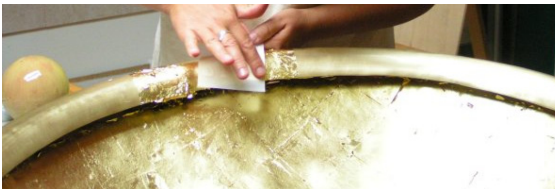
Figure 11: Gilding of a fountain element
